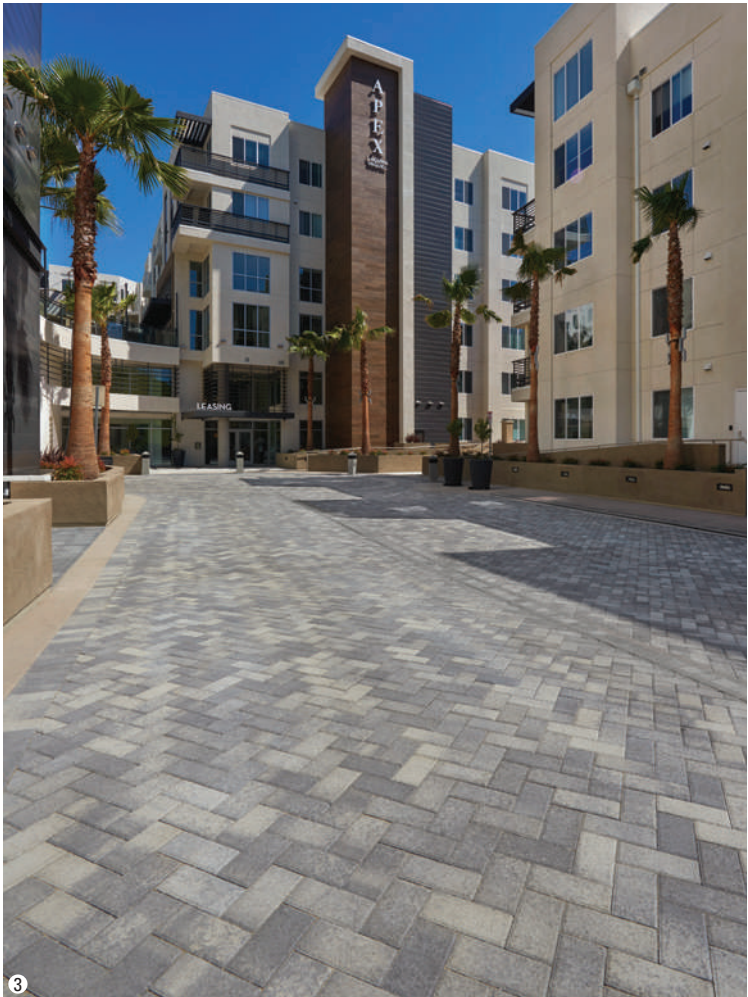
1. Cream-Brown-Charcoal Holland installed in a running bond pattern with a solid Mocha Holland border at the landscape edge. 2. Tuscan Holland installed in a running bond pattern. 3. Holland in Gray-Charcoal installed in a 45 degree herringbone pattern. Note: This stone was manufactured at 80mm due to site conditions and anticipated traffic loads. 4. Holland in Gray-Charcoal installed in a running bond pattern. Border is Holland Gray-Charcoal in a soldier course.
