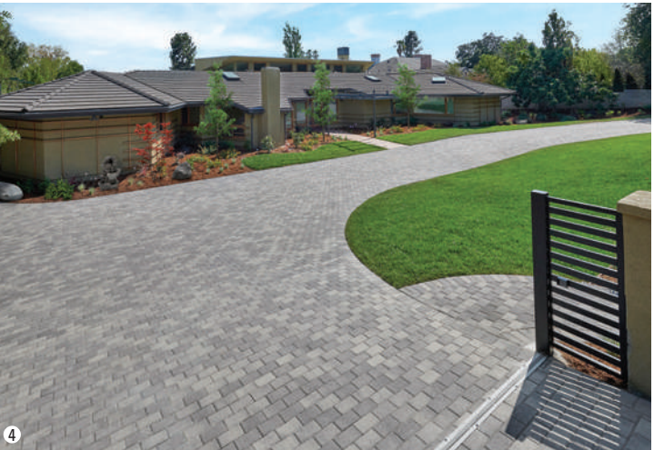
1. Cream-Brown-Charcoal Holland installed in a running bond pattern with a solid Mocha Holland border at the landscape edge. 2. Tuscan Holland installed in a running bond pattern. 3. Holland in Gray-Charcoal installed in a 45 degree herringbone pattern. Note: This stone was manufactured at 80mm due to site conditions and anticipated traffic loads. 4. Holland in Gray-Charcoal installed in a running bond pattern. Border is Holland Gray-Charcoal in a soldier course.
