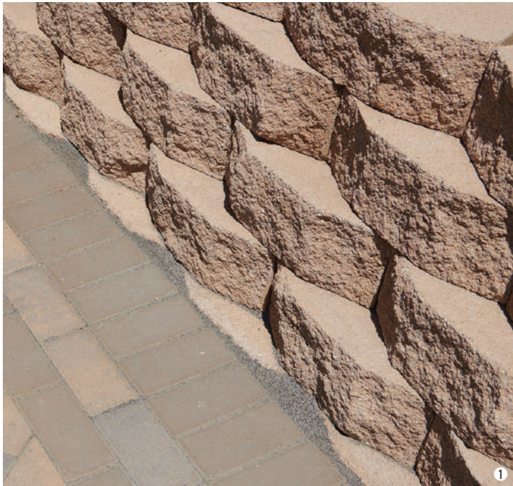
1. Tan 16" Planter Wall in a common bond pattern. Pavers are Courtyard Stone in Tuscan installed in a 45 degree random ashlar pattern. Border is Holland Mocha soldier course, Holland Tuscan in a running bond and Holland Mocha in a running bond. 2. Tan 16" Planter Wall in a common bond pattern. 3. Charcoal 16" Planter Wall in a common bond pattern. 4. Tan 16" Planter Wall in a common bond pattern. Pavers are Courtyard Stone in Tuscan installed in a 45 degree random ashlar pattern. Border is Holland Mocha soldier course, Holland Tuscan in a running bond and Holland Mocha in a running bond.
